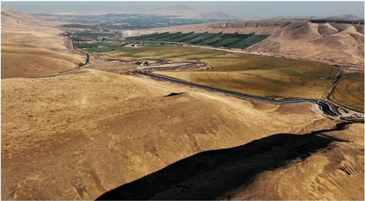
This view shows the Dennis Road possible wind turbine tower location east of Weber Canyon looking northwest towards Benton City. Courtesy Bruce Bjornstad
